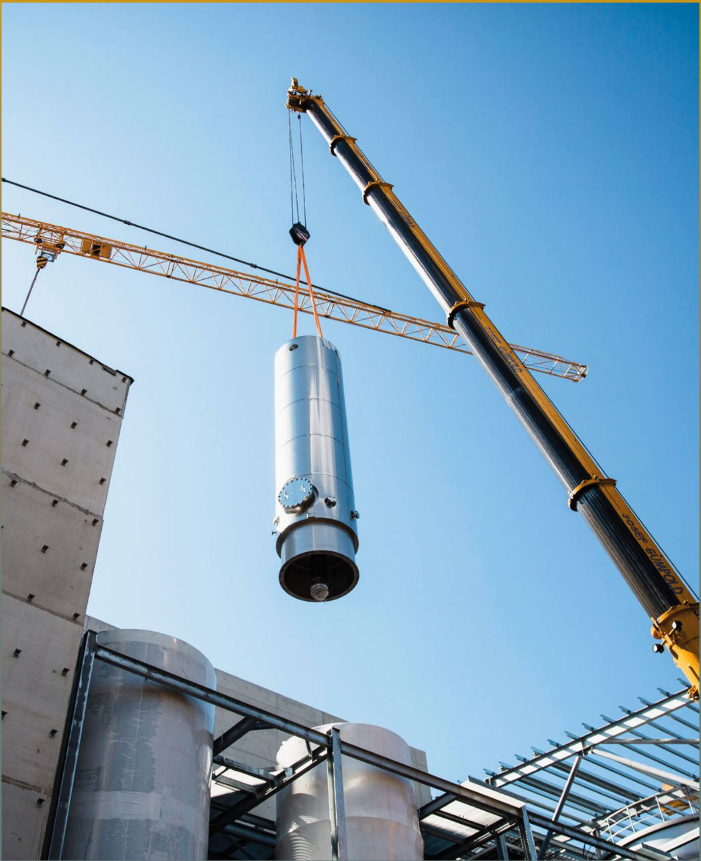
Above: TowerBrook's investment supported the installation of a Cleaning-In-Place (CIP) facility at AustroCel Hallein
